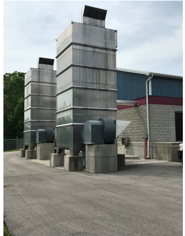
Air Strippers for the removal of the VOC chemical Tetrachloroethylene "PERC" have been working now for 6 years.
