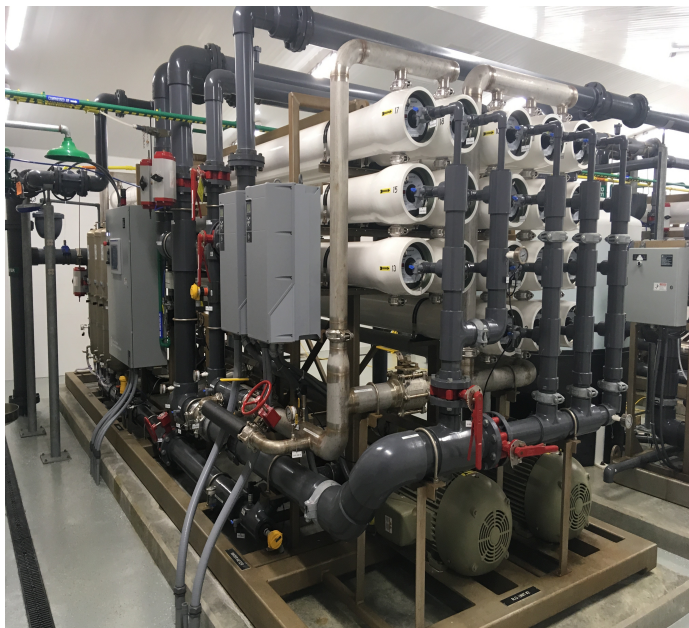
Reverse Osmosis 1,100 GPM Water Treatment
